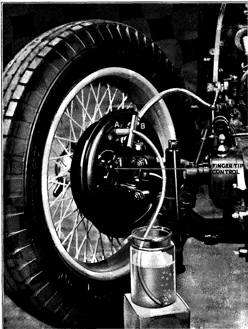
Illustration No. 18. —Bleeding part of the braking system ; note the special tool provided for the job.
